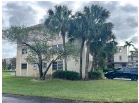
Building left side view.
