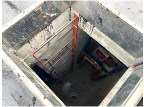
Reinforced concrete roof deck.
