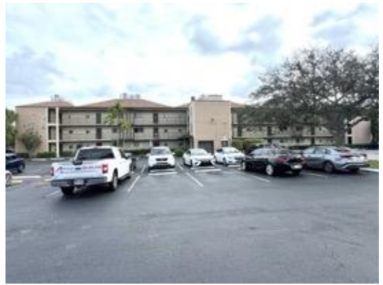
Building front view.
