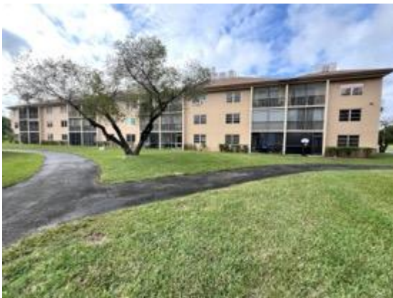
Building rear view.
