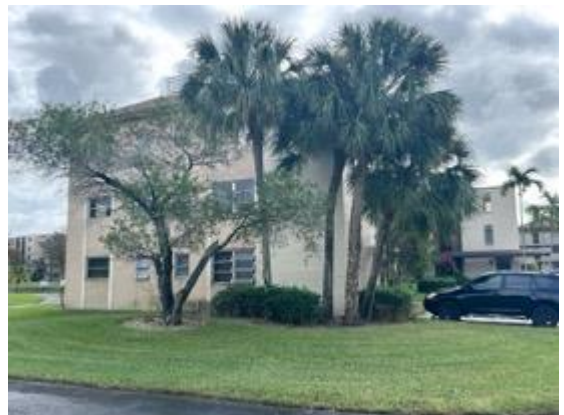
Building left side view.
